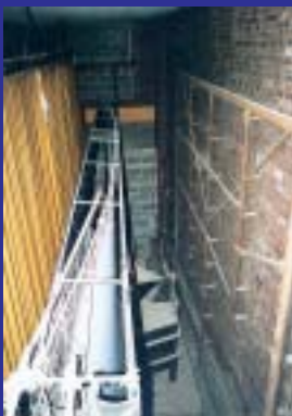
An original wooden wall mounted screen frame behind an updated curved replacement - at the Curzon Cinema, Clevedon, UK
